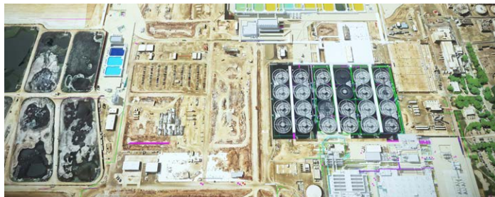
Regional San initiated the decade-long EchoWater facility upgrade to provide safe and reliable treated water for recycled water use.
